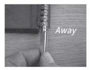
12) Lay the door panel back in the frame. You may pull cable to retract the latch while doing this.
